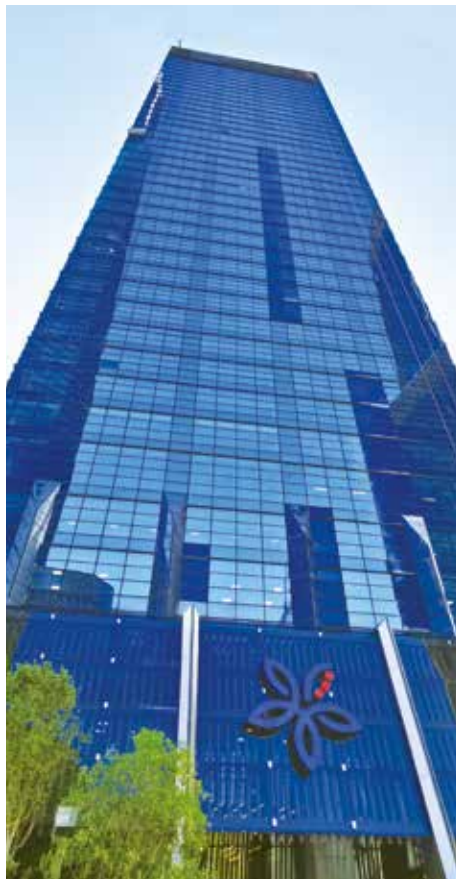
▲ Our new headquarters, Menara Affin Bank at Tun Razak Exchange.
