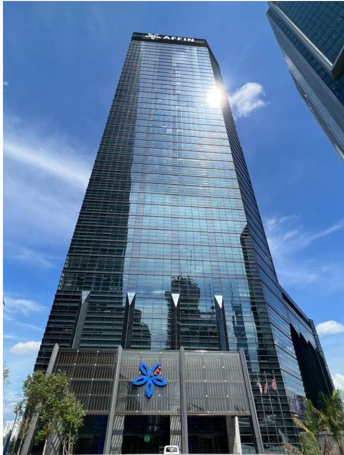
Best Project Award – Building (Major Category) by Construction Industry Development Board (CIDB) for Menara AFFIN @ TRX
